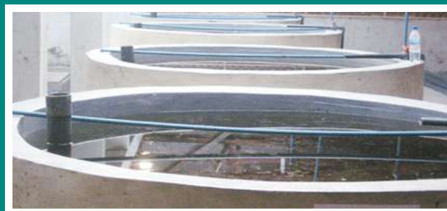
Circular concrete tank for shrimp hatchery at NIOMR, Badore, Lagos State
