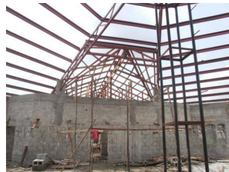
EDC under construction
