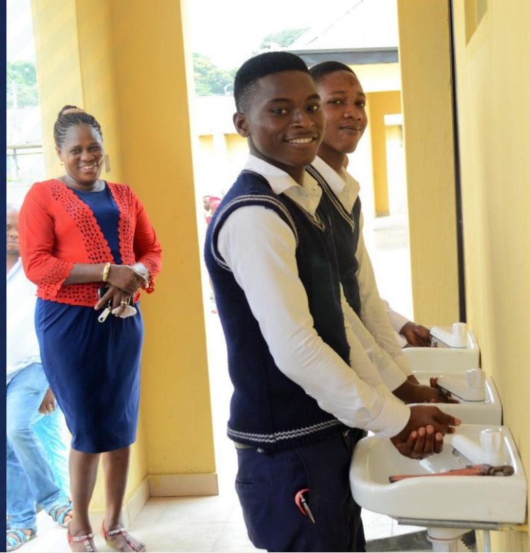
Students at Government Technical College Port Harcourt, Rivers State, use their newly-installed toilet facilities while their principal, Mrs Rosemary Adooh (in a red jacket) looks on
